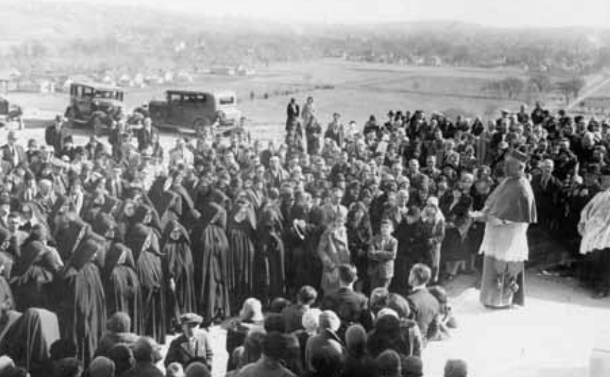
Groundbreaking ceremony on Oct. 5, 1929, for construction of Heelan Hall with Bishop Edmond J. Heelan, Sisters of Saint Francis and Mother Mary Dominica Wieneke, foundress of Briar Cliff.
